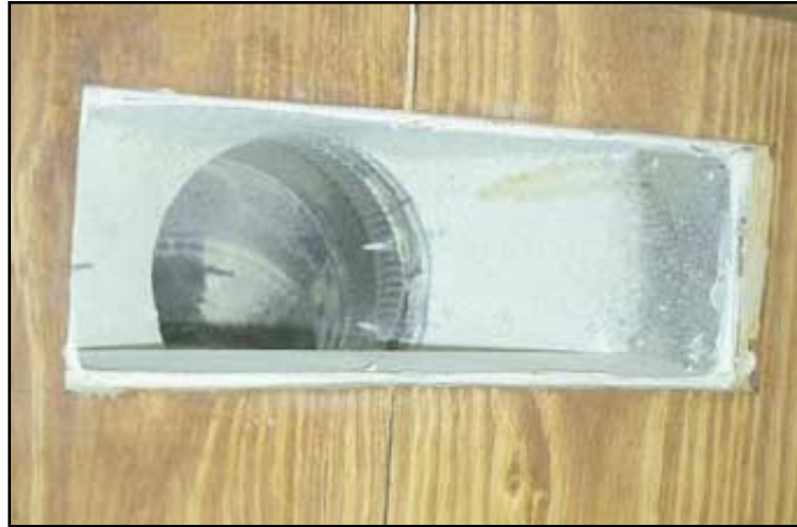
A supply boot is caulked to the floor to reduce leakage.
