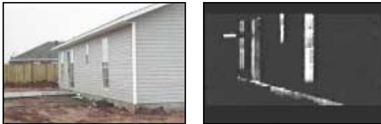
Infrared picture of slab heat loss with insulation under slab.
