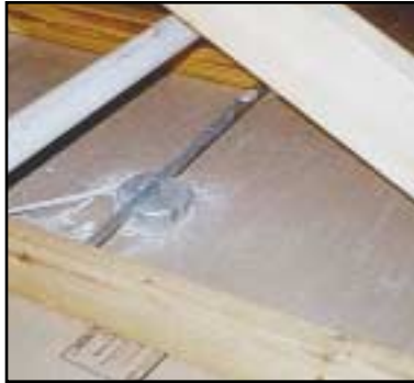
Sealed with caulk
