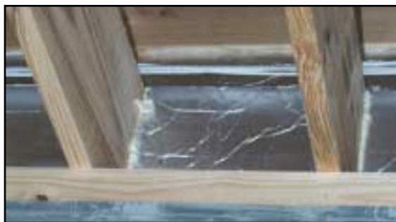
Joist cavity is blocked and sealed to prevent attic or outside air from entering between floors.
