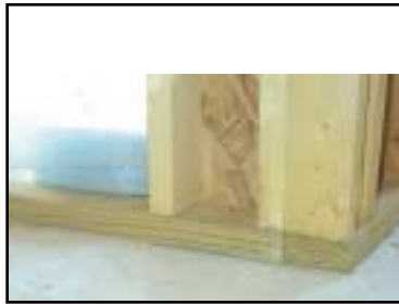
Sealing bottom plate with foam sill-sealing product
