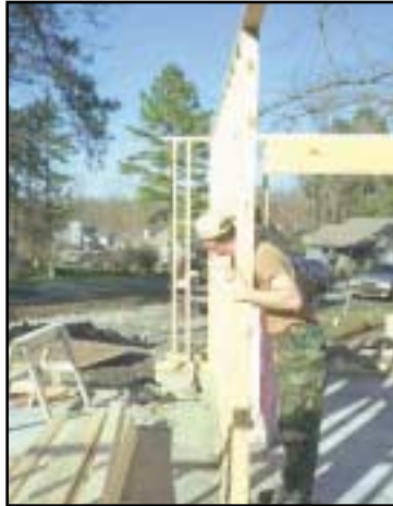
Framing the wall
