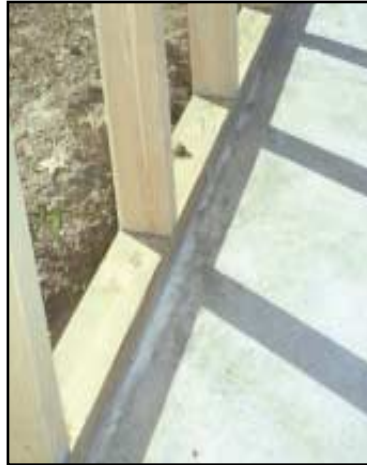
Exposed foam will be covered with drywall and molding
