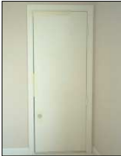
The attic access door should be treated as an exterior door with good weather-stripping, a threshold and a secure latch. Best practice would also include adding some rigid insulation to the backside of the door
