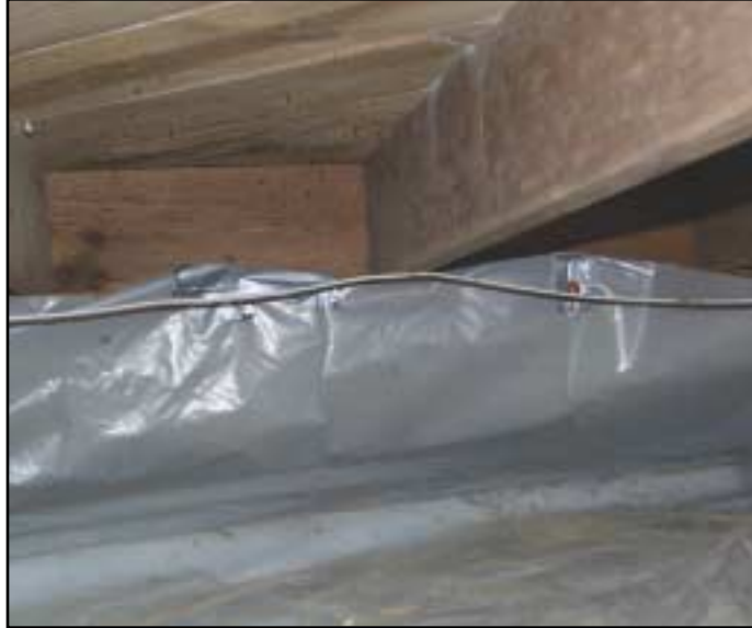
Crawlspace ground cover
