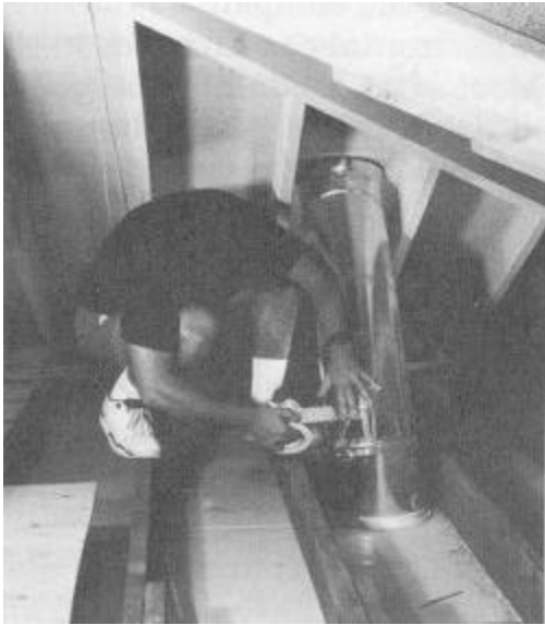
Figure 2 --The basic Solatube kit includes one straight section and two elbows. The 10-inch diameter tubes fit easily between rafters and joists.
