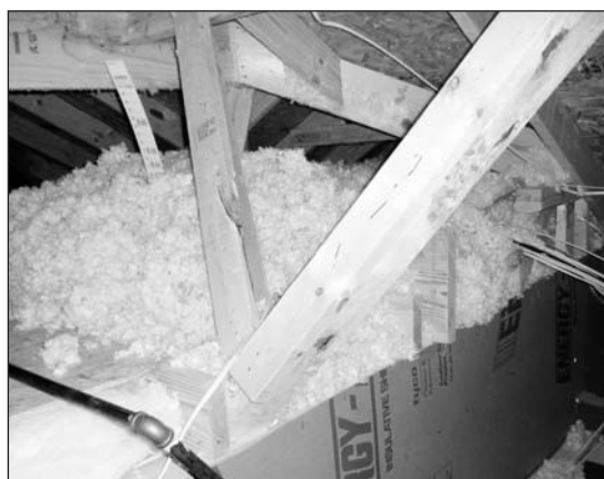
The 8ft by 10ft raised area shown is a Grade III installation at best; 10% of the area clearly is short of the indicated thickness by 30% or more.
