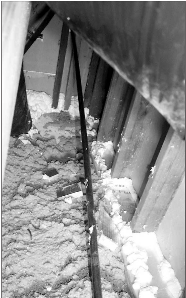
It's important to seal cavities connecting the house to the attic. Foam was used for sealing small holes and cracks at building component intersections.
