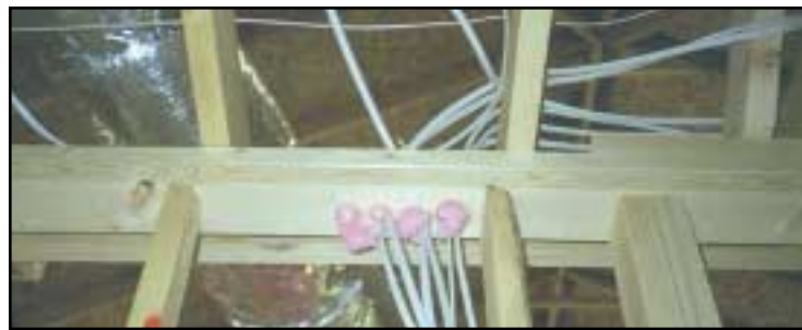
Foam all penetrations in the top plates.
