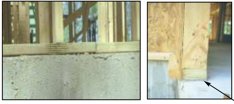
Seal areas between wood and concrete with foam sill seal.
